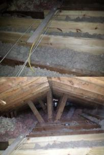
\* There is evidence of past rodent and/or squirrel activity on the insulation (trails, tunnels, droppings, etc.).
