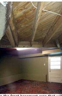
\* There is some light surface mold visible on the floor joists and sub flooring in the front basement area that will need to cleaned with a bleach solution and dried out for health and welfare.
