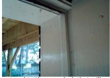
\* There is water damaged and rotted wood trim at the exterior doors of the basement and to the rear deck that will require repair, caulk and paint.
