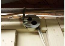
\* There is an open gap in the AC coolant line visible in the front unfinished basement that will need to be sealed to prevent condensation from dripping off the line in the cooling mode.
