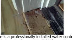
S-2,14.....\* There are several significant patches of the block foundation walls and there is a professionally installed water control system along the exterior walls the result of settling and moisture penetration into the basement of this home. Repairs were professionally done and a warranty should be included for the system and work. Recommend monitoring for additional cracking and any possible moisture penetration.
