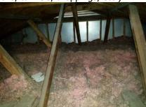
A-9,10.....\* There are water stained roof sheathing boards around the roof penetrations from past leaks that should have been repaired when the roof shingles were replaced, the areas should be monitored during heavy storms to ensure leaks are not active as there was no moisture at the time of inspection. Boards may need to be replaced when the shingles are next replaced.
