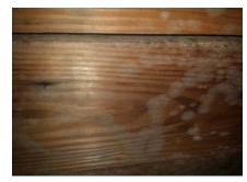
The ventilation for this attic is insufficient for current construction practices and could cause roof shingles to curl and lift prematurely due to the build up of heat in the attic. A ridge vent would be the best option for this roof type. Recommend adding ridge and more soffit vents when the roof shingles are next replaced which would eliminate the need for the surface and gable vents. There is a loose screen on a gable vent that needs immediate repair.
